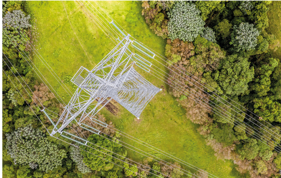
Transmission tower in the Filandia municipality, part of the Armenia project between the Quindío and Risaralda departments
