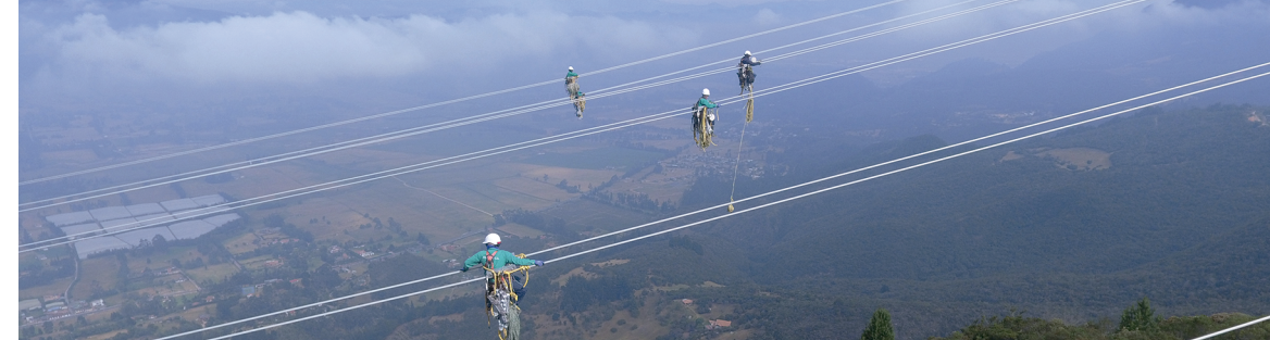
Transmission line maintenance at Guavio-Circo
