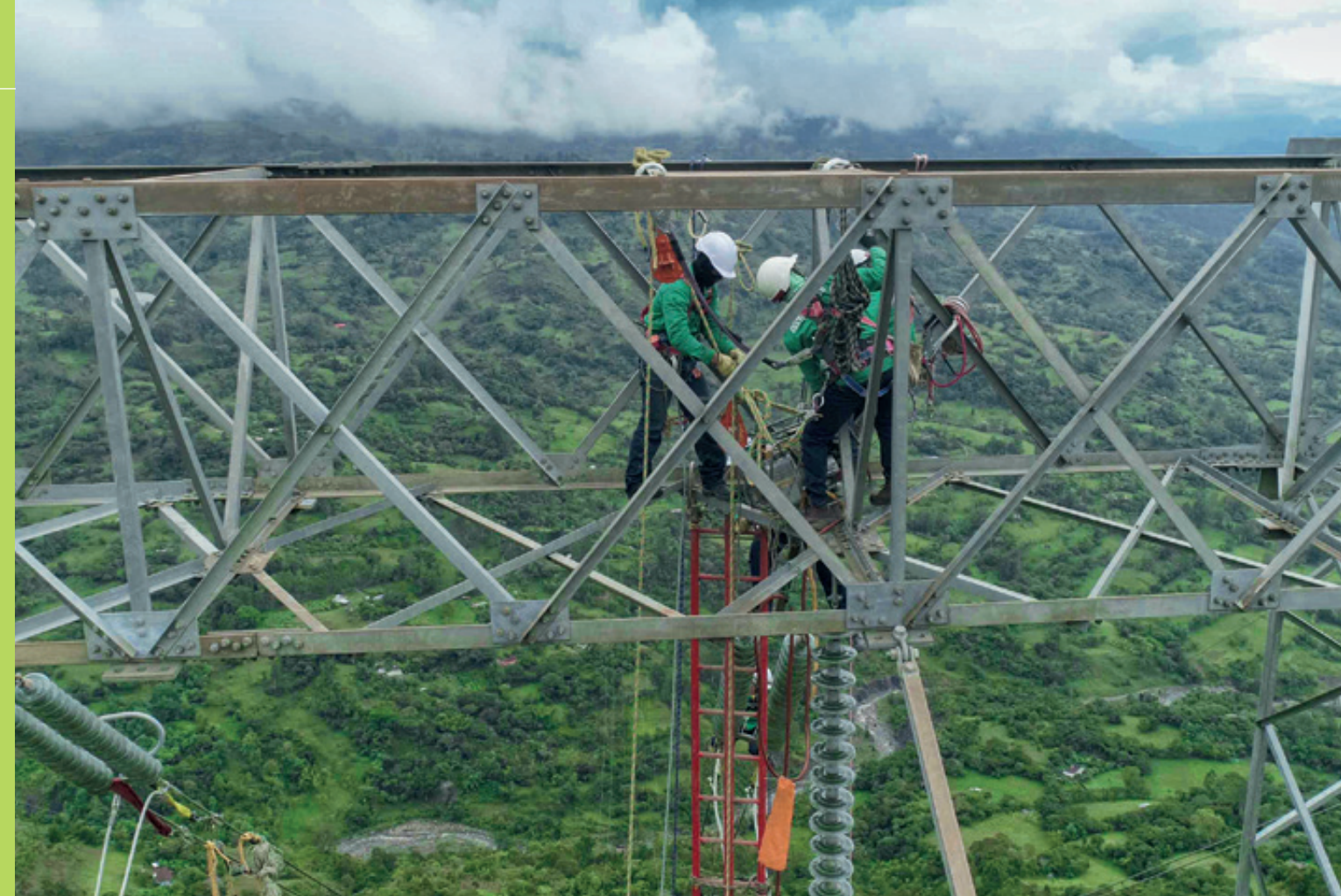
A lineman spends an average of eight hours a day working at heights during maintenance of the transmission lines; Tower 77 of the Guavio, Circo line
