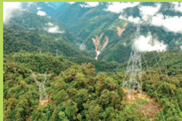
After a lot of hard work, the tower was raised, which enables the transportation of electric energy to southern Colombia
