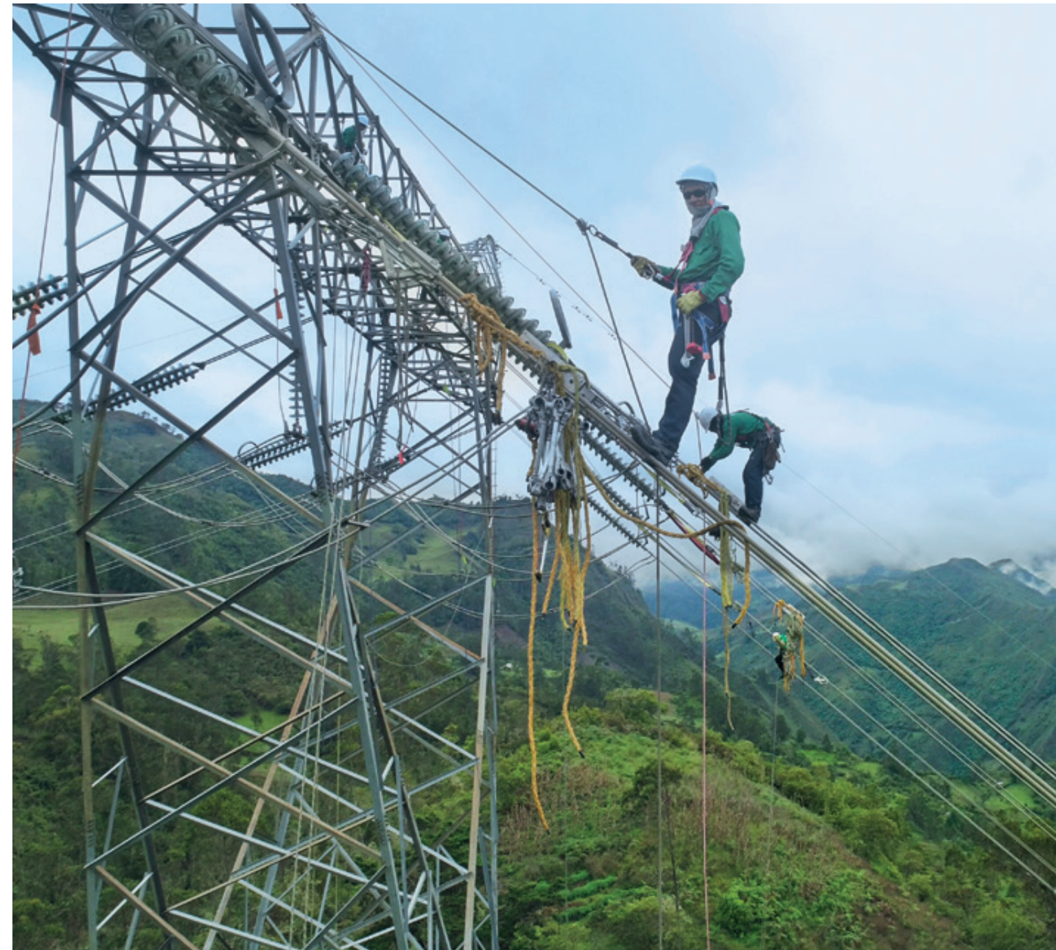
Maintenance of transmission lines at Circo-Guavio, tower 77
