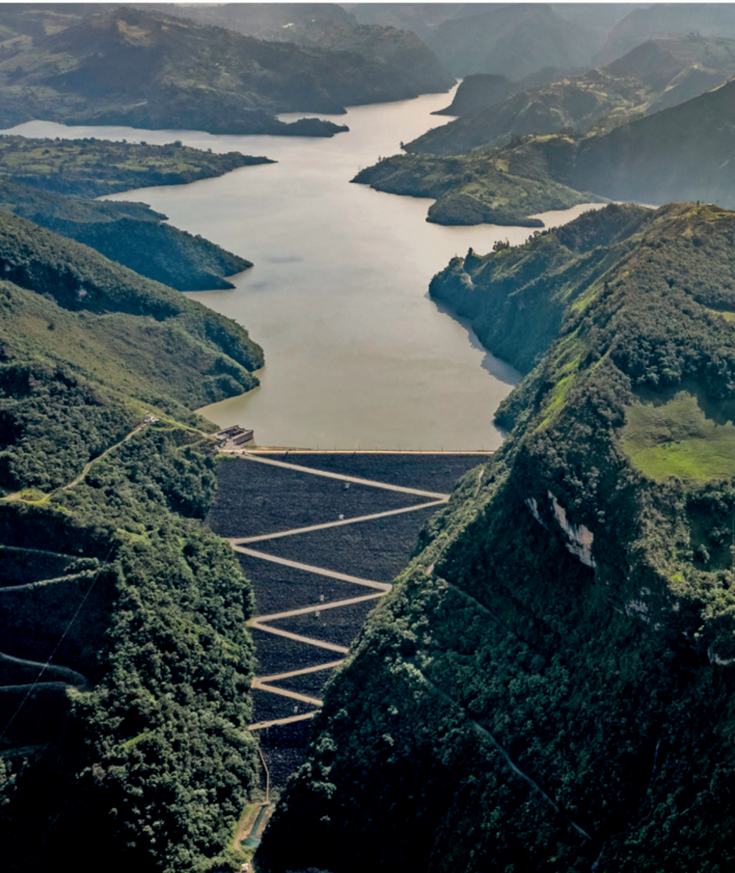
Guavio dam owned by Emgesa
