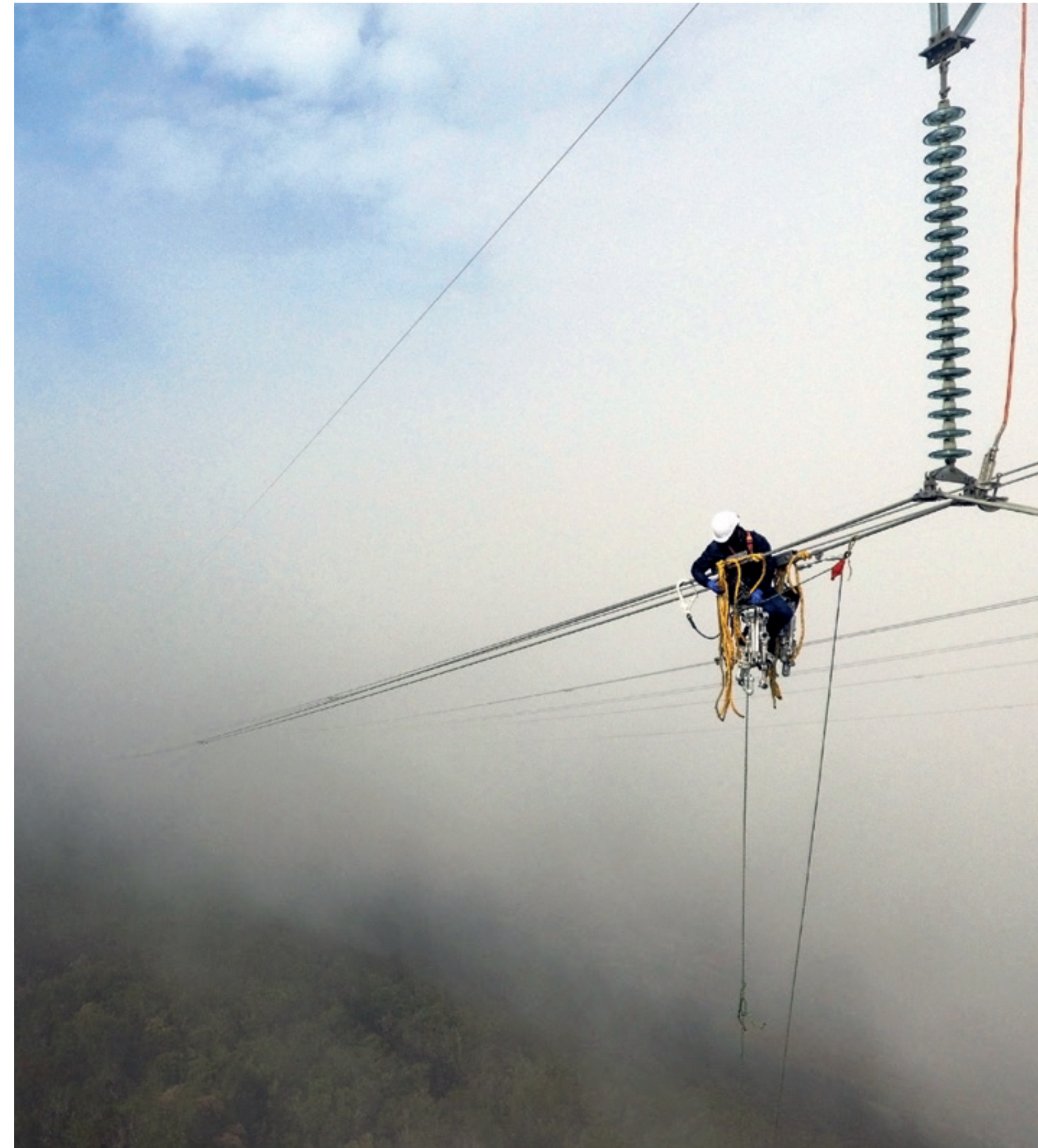
Maintenance work on our transmission lines in Guasca, Cundinamarca
