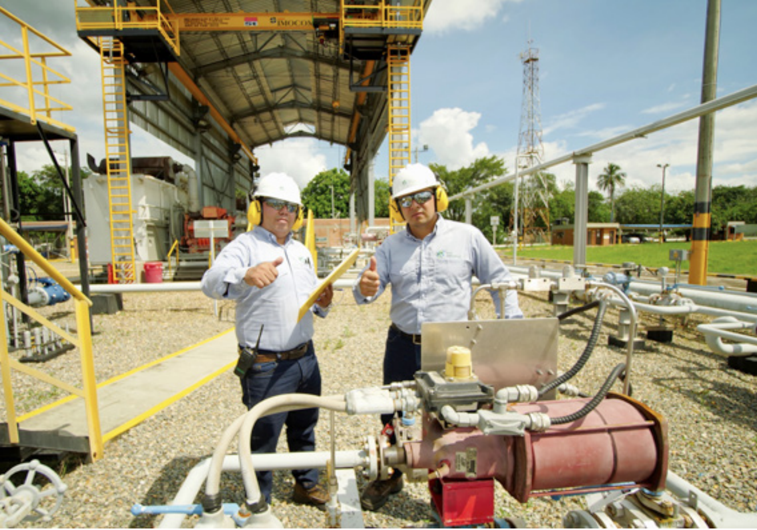
TGI engineers at the Mariquita Station, Tolima
