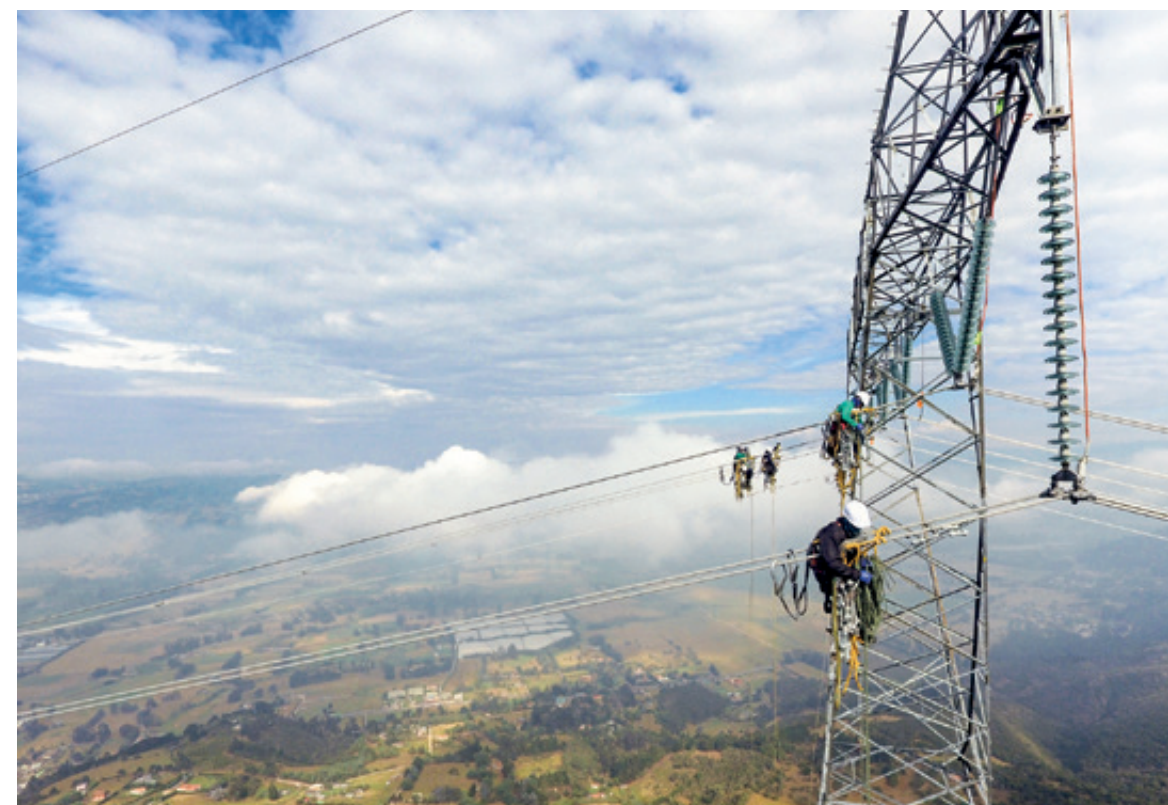
Maintenance work at our transmission lines in Guasca (Cundinamarca)
