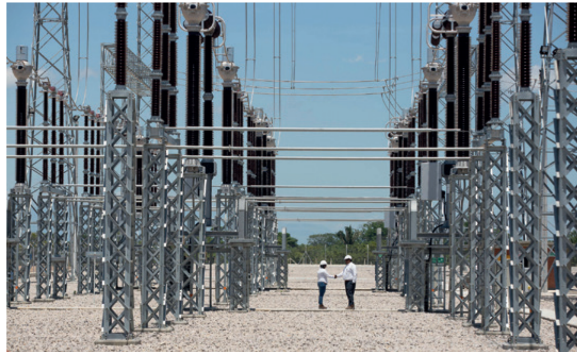
Our substations have state of the art technology that enhanced service quality
