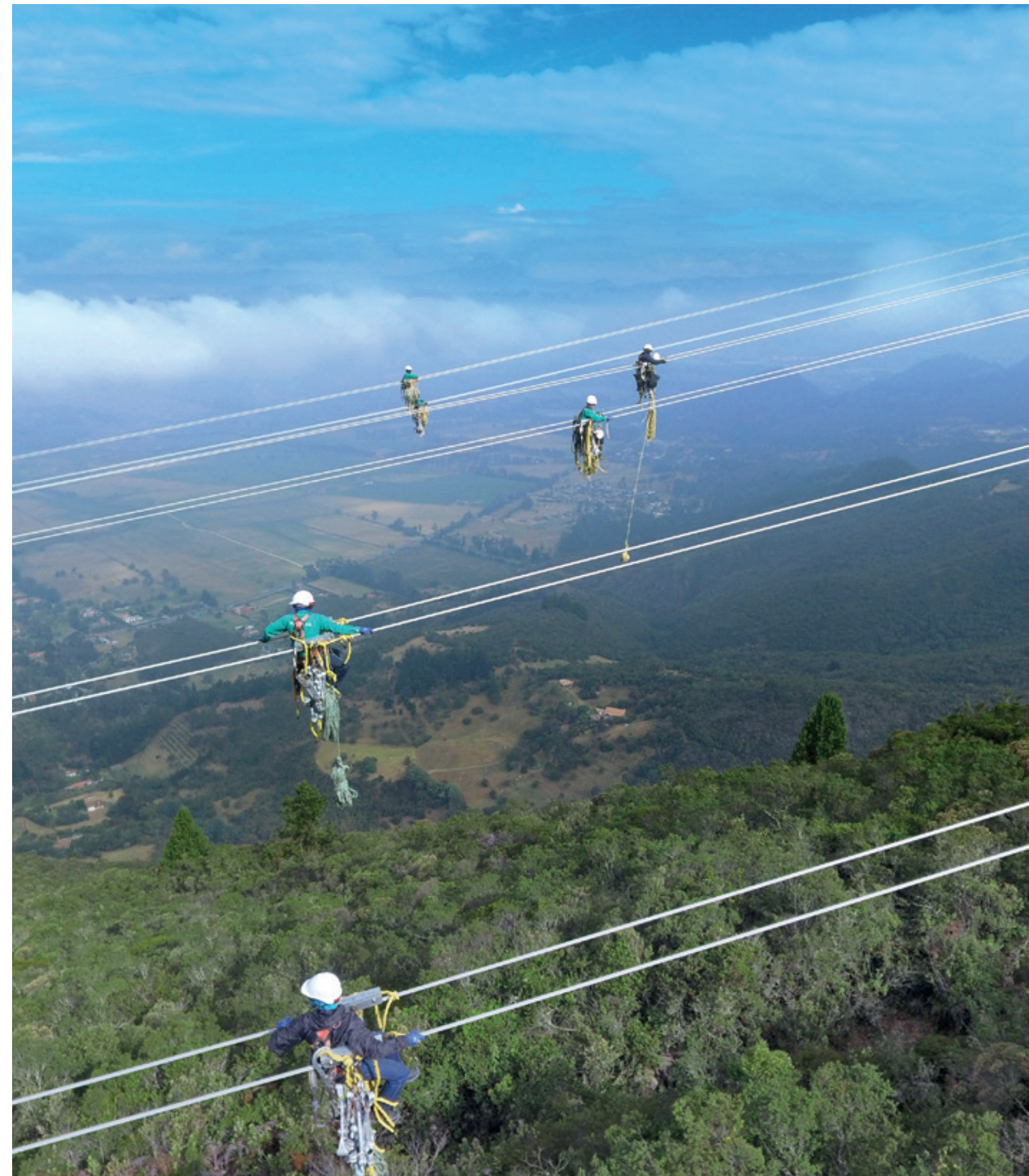
Maintenance work on our transmission lines at Guavio-Circo in Guasca, Cundinamarca
