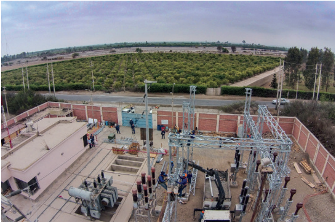
Electro Dunas infrastructure in Peru
