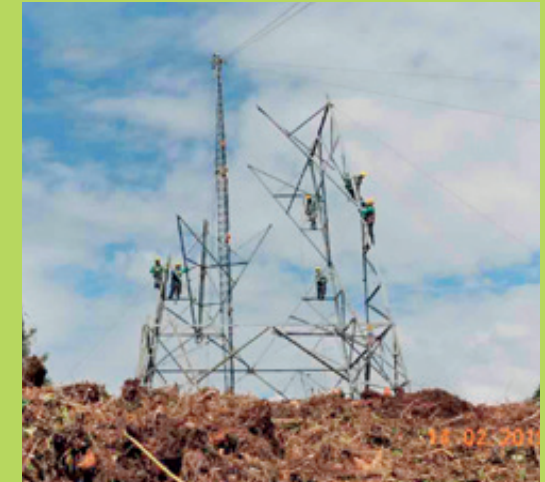
Construction work of tower 309, second section of the Tesalia - Alférez project in Pradera, Valle del Cauca
