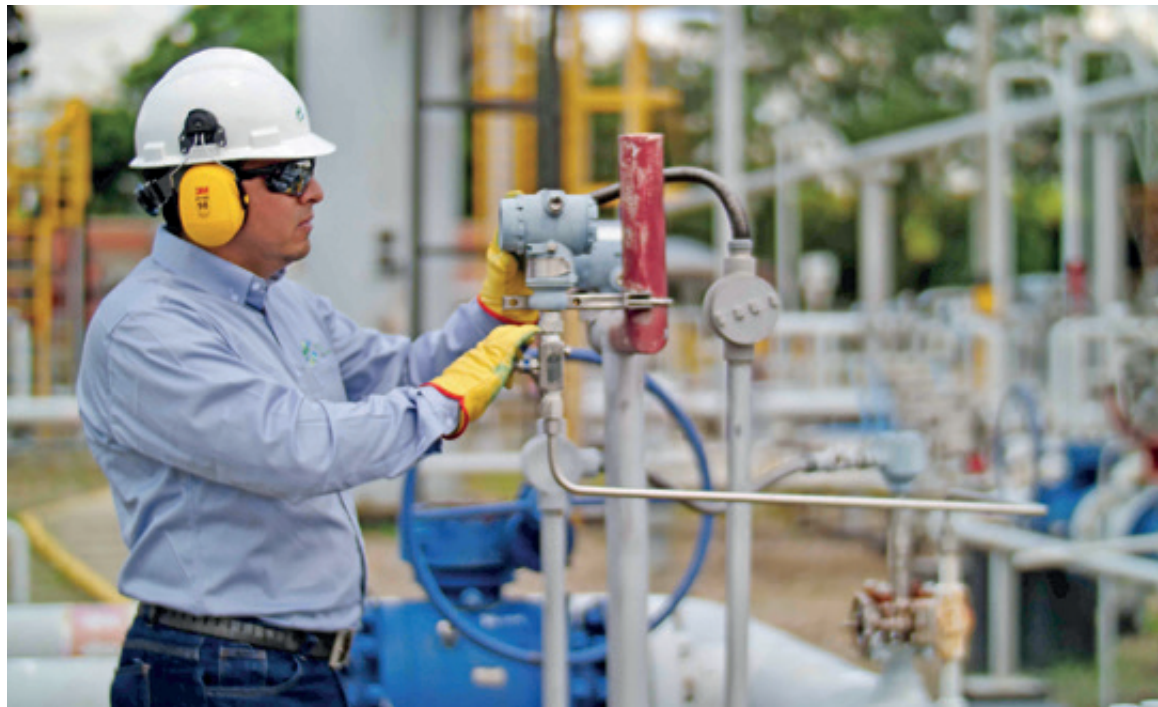
TGI employees at the Mariquita gas compression station in Tolima
